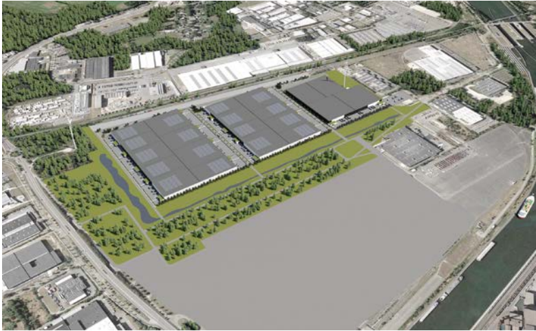
Genk Green Logistics Redevelopment zone B
