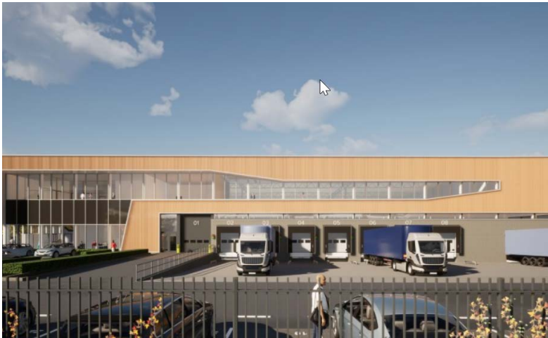
's-Hertogenbosch Rietvelden Commercialization built-to-suit logistics project
